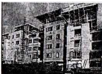
Building construction for several apartment blocks
