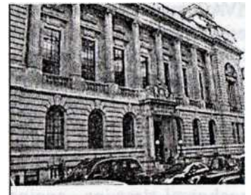
Institution of Civil Engineering headquarters in London
