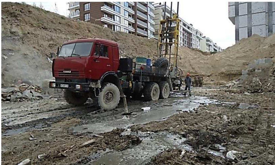
Fig. 5. Production work on the fixing soil-cement elements using drill-mixing technology
