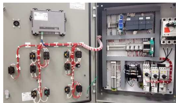
Fig. 4. Control system with PLC placed inside the rack cabinet with DIN rails
